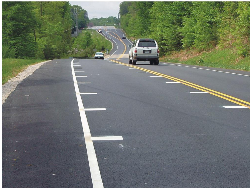
Figure 22. Optical Speed Bars on South End of Lee Chapel Road Installation (Virginia, US). Top: View Looking North. Bottom: View Looking South. Source: Arnold and Lantz (2007).
